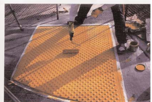
SAFTI-TRAX Application on Ramp
